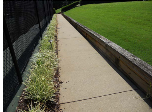
Wood Retaining Wall
