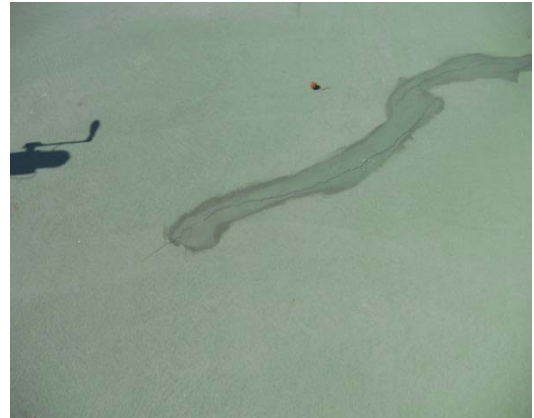
Cracked Playing Surface
