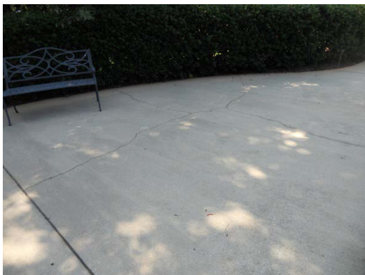
Cracked Flatwork Outside Tennis Court
