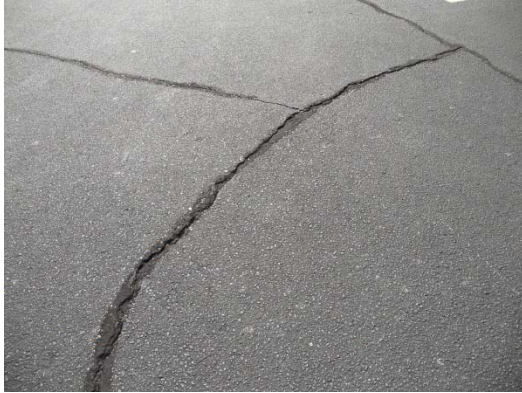
Asphalt Cracking
